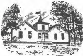
Jacob's Graded School, Hall Township.
